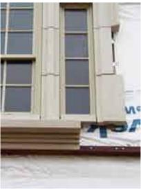
Steel beams offer support for the sill as it is prepared for mortaring.
